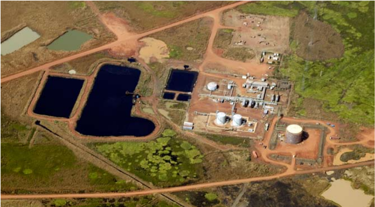
An aerial view of the Unity Oil Field operated by the Greater Nile Petroleum Operating Company (GNPOC), Bentiou, Sudan, 5 November 2008. UN Photo/Tim McKulka
